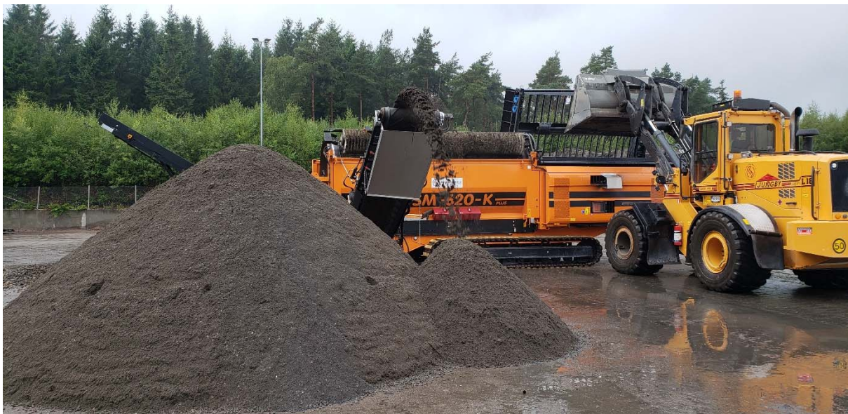
PFAS contaminated soil being treated with RemBind® in Sweden
