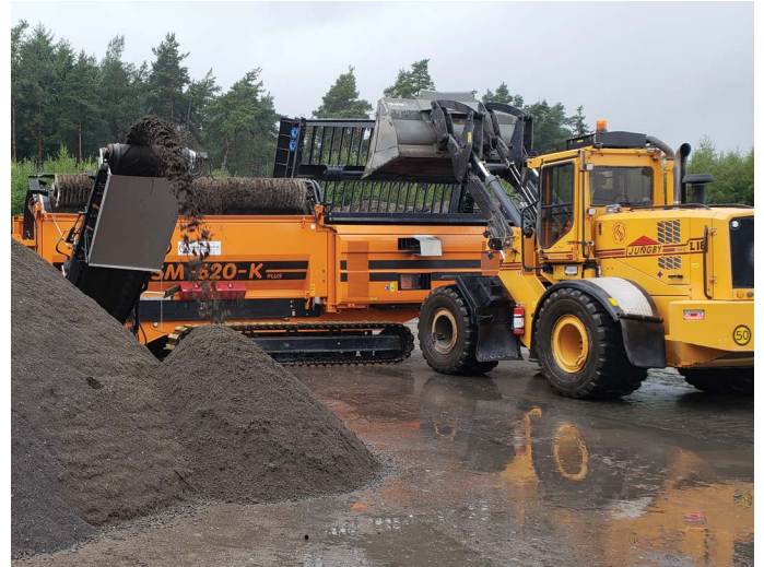
RemBind being applied to treat PFAS soil in Sweden
