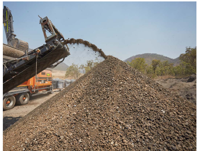
RemBind being applied to treat PFAS soil in Australia
