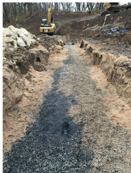
Groundwater Remediation (Permeable Reactive Barrier)
