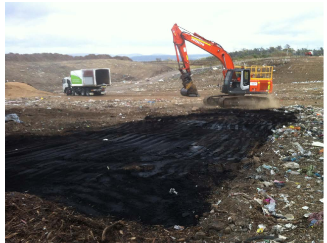
The finished RemBind cap on the burial pit
