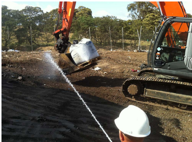
Adding RemBind to form the base of the burial pit
