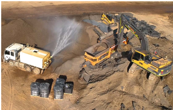
Soil Treatment Site
