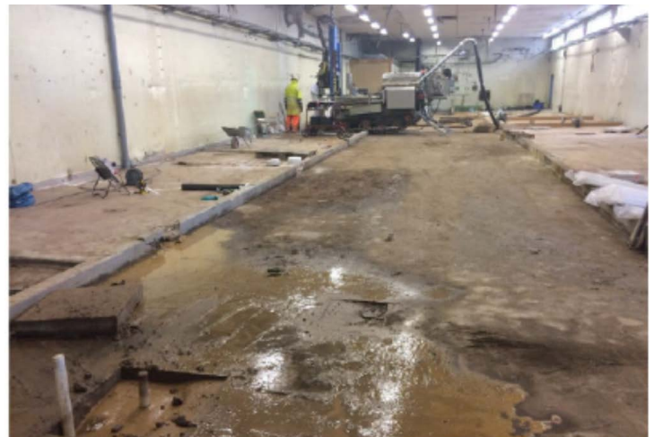
Demolition of Former Metal Plating Factory
