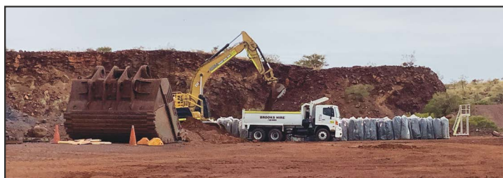
Figure 4: Mixing RemBind® into Soil with Excavator
