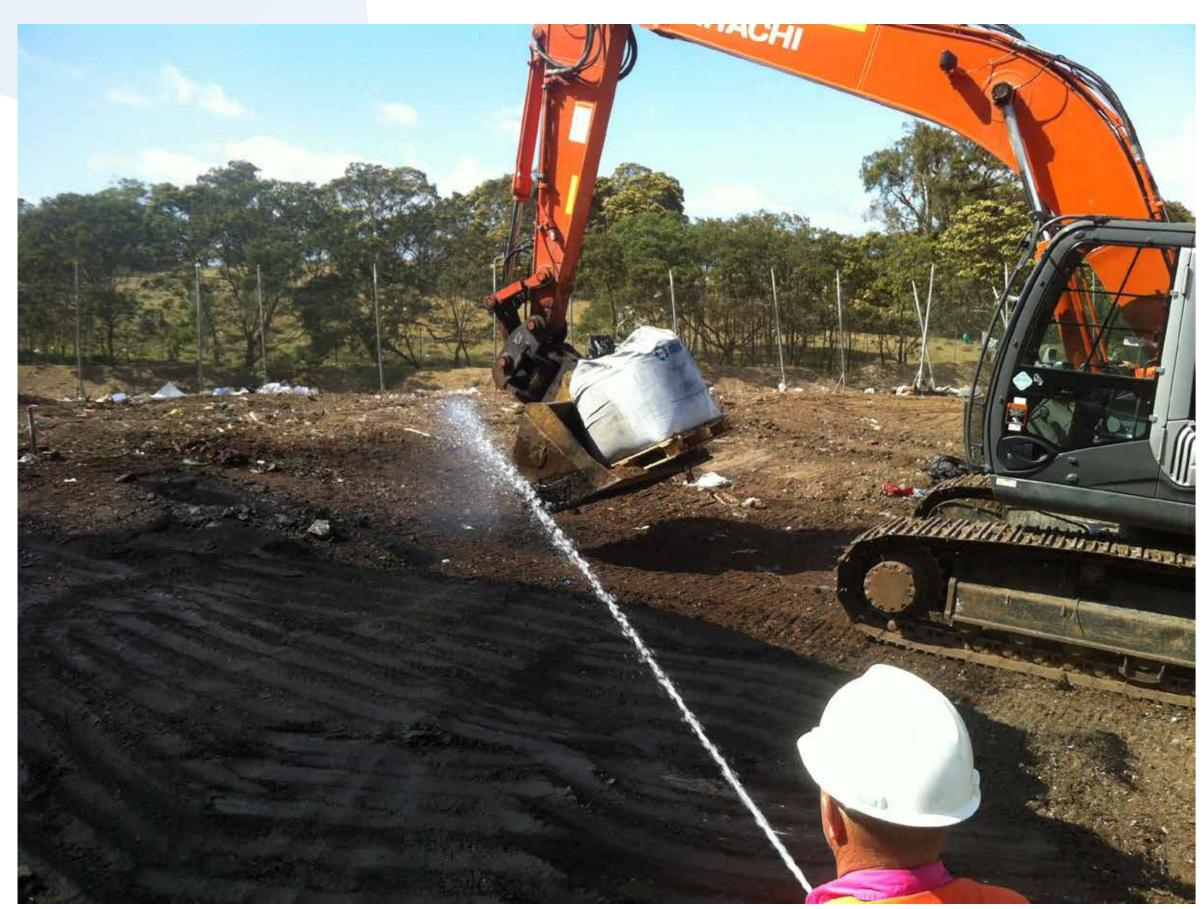
Figure 1: PFAS impacted soil being treated with RemBind
